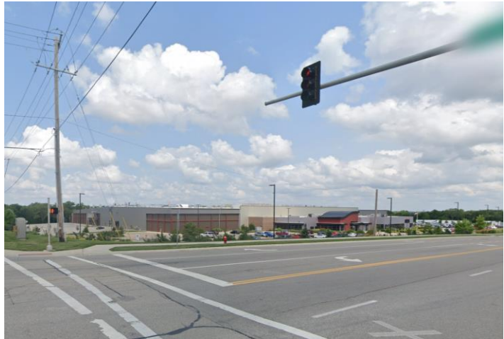
Existing Reser's Plant, View from SE 6 th and Croco Rd.
