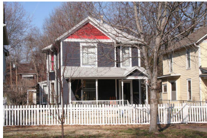
1115 SW Western. East elevation. 03/28/2013. KSHS.
