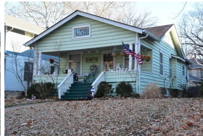
116 SW The Drive. Topeka, Shawnee County, Kansas. View NE. 01/09/2019. Finch, Brad.
