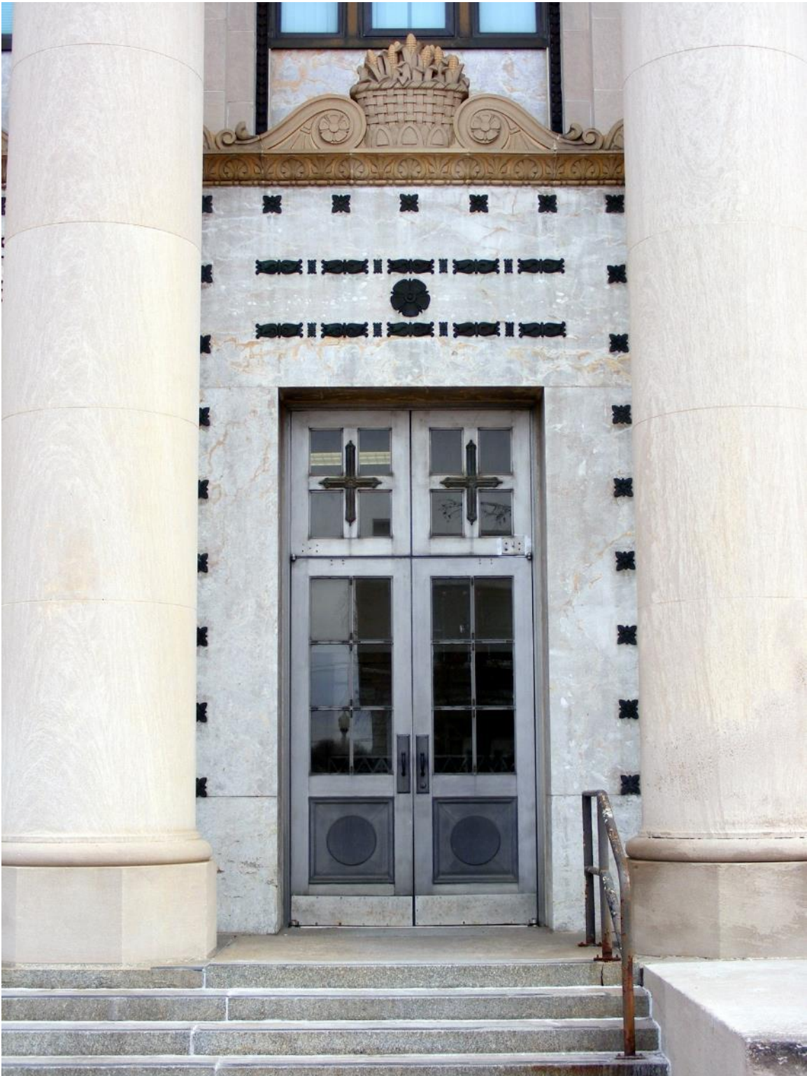
KS_Shawnee County_United States Post Office and Court House_0004
