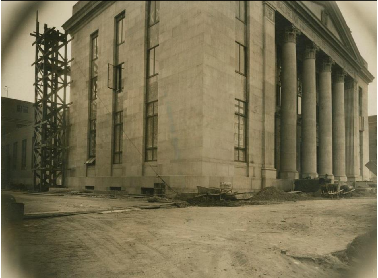
Figure 3. A construction progress photograph from November 1, 1933 shows the building's original casement windows.
