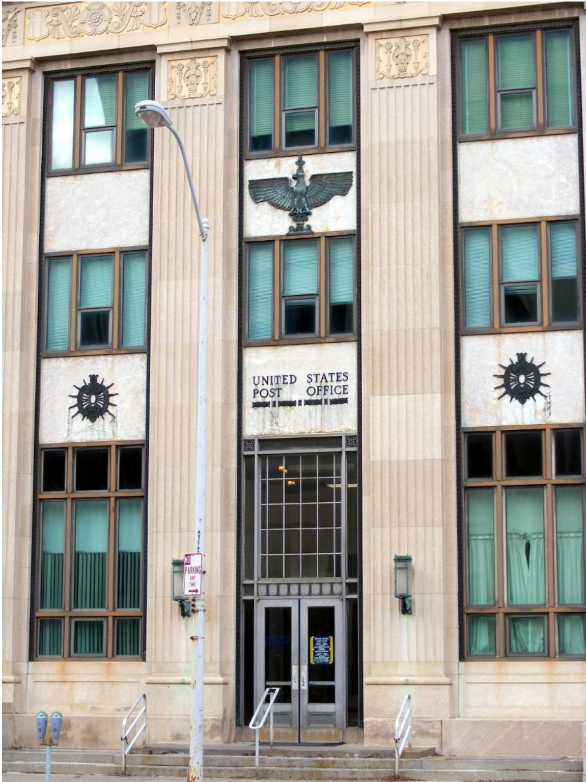
KS_Shawnee County_United States Post Office and Court House_0006
