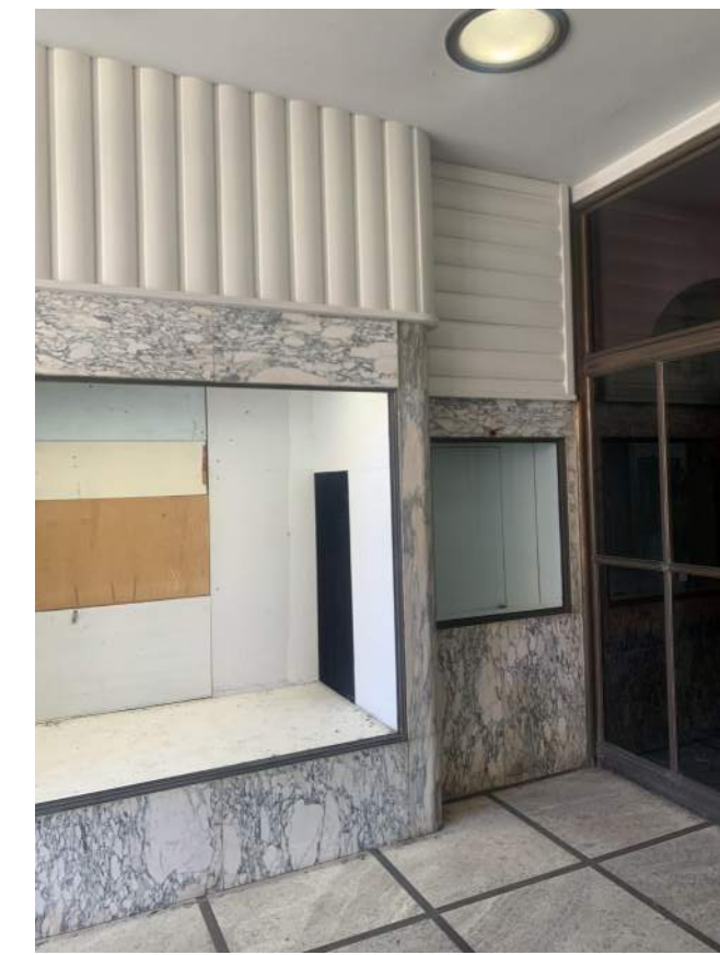
14 SOUTH-WEST CORNER Future Vestibule
