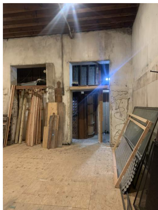
4 SOUTH-EAST CORNER Future Barber Shop
