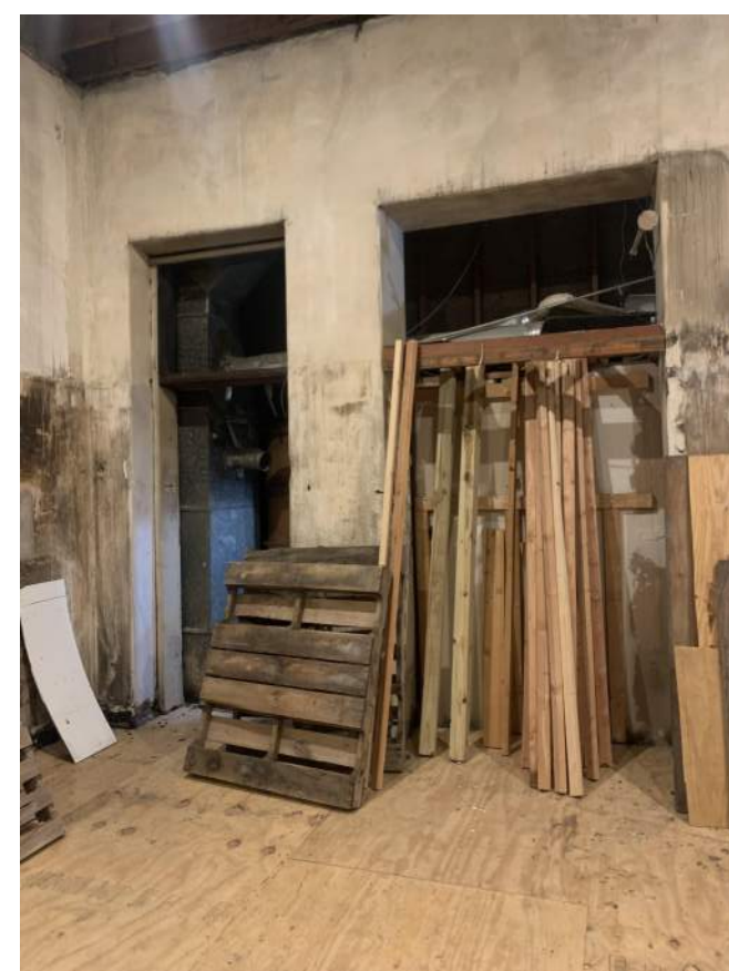
3 NORTH-EAST CORNER Future Barber Shop
