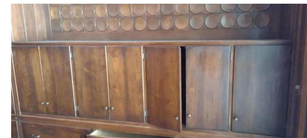
21 MID SECTION Existing Cabinets
