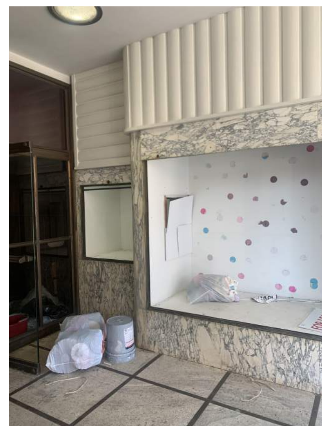
16 NORTH-WEST CORNER Future Vestibule
