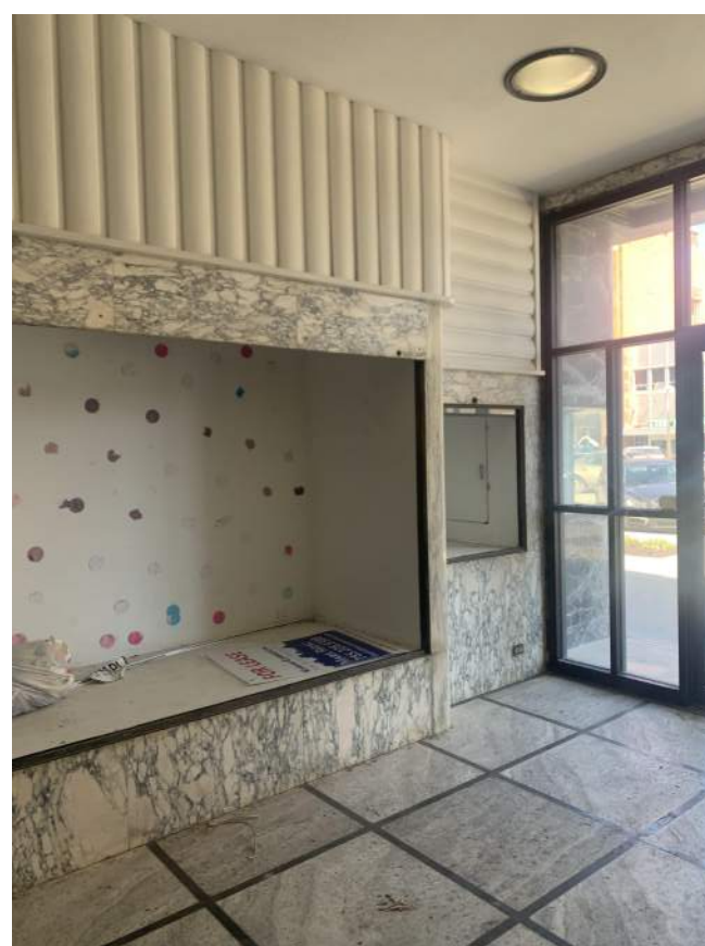
15 NORTH-EAST CORNER Future Vestibule
